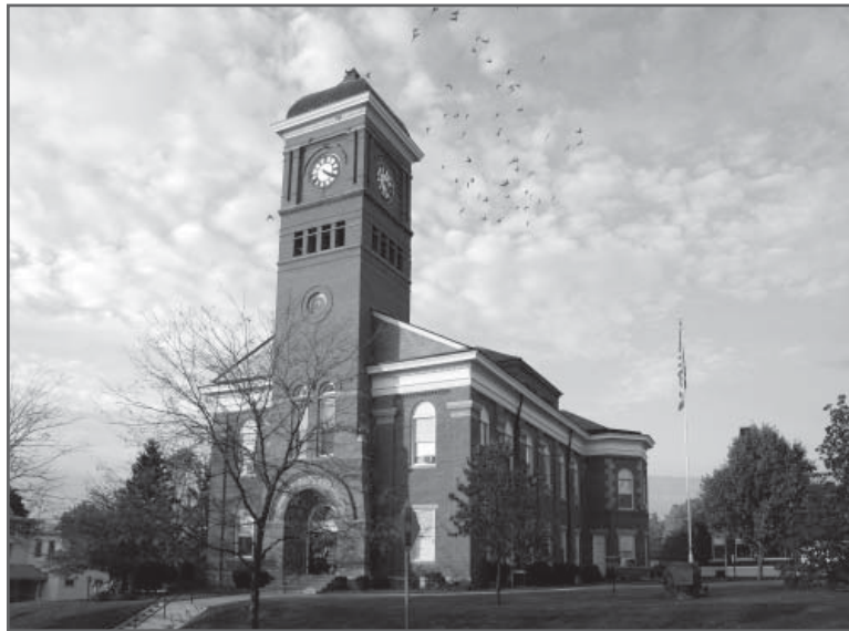
Morrow County Courthouse Mount Gilead
